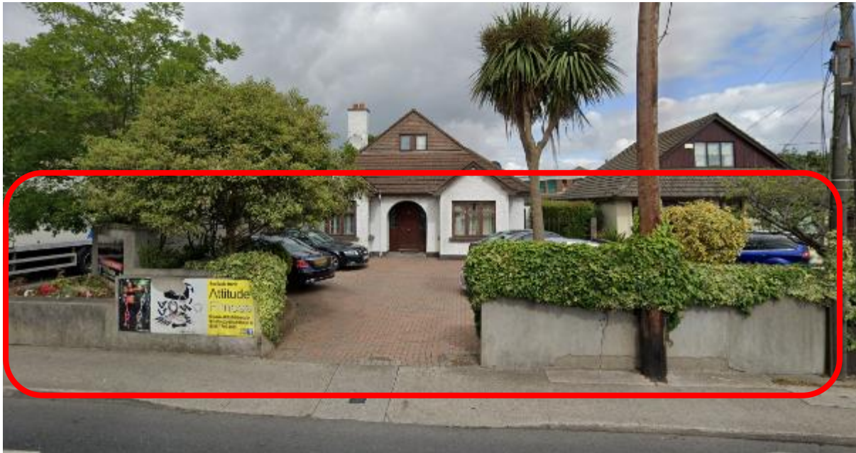
Figure 3.4.7: Existing Street View at Maria Philomena, Mornington Park, Malahide Road (Image Source: Google )
