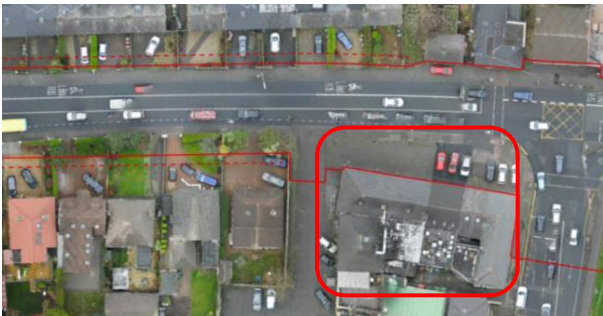
Figure 3.6.14 Existing aerial view of the Goblet Bar and Lounge
