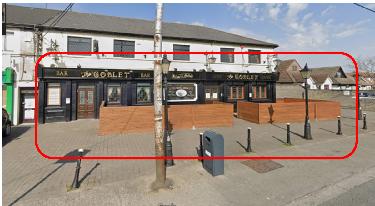
Figure 3.6.15 Existing Street View of the Goblet Bar and Lounge (Image Source: Google )
