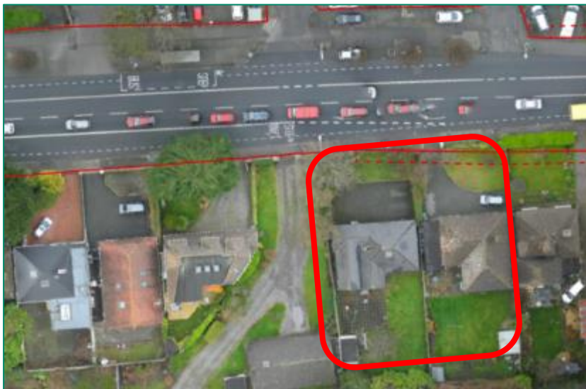
Figure 3.4.3: Existing aerial view at Northern section of Mornington Park, Malahide Road
